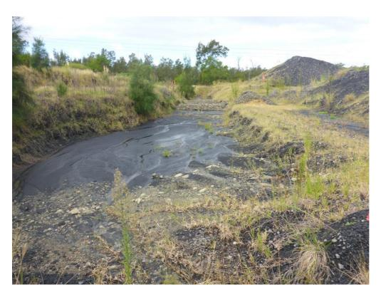
Photo 6 Coal Material in drain should be removed
